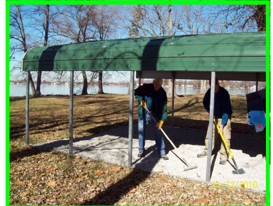
Ron and Dan hard at work, leveling the gravel
